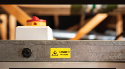
Warning and identification labels for conduit and trunking enclosures that protect and hide cabling.
